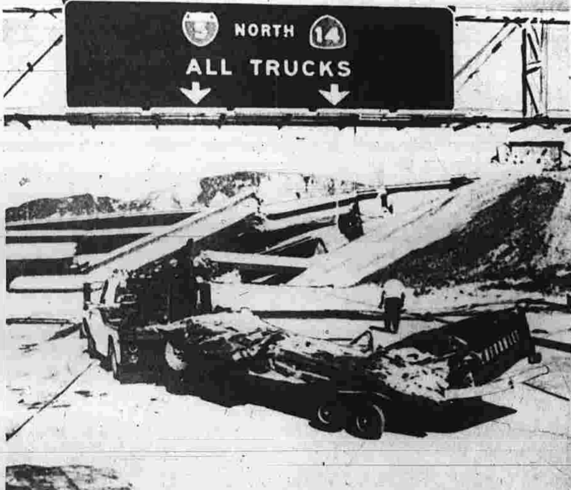
Tow truck hauls away wreckage of truck smashed when overpass fell
