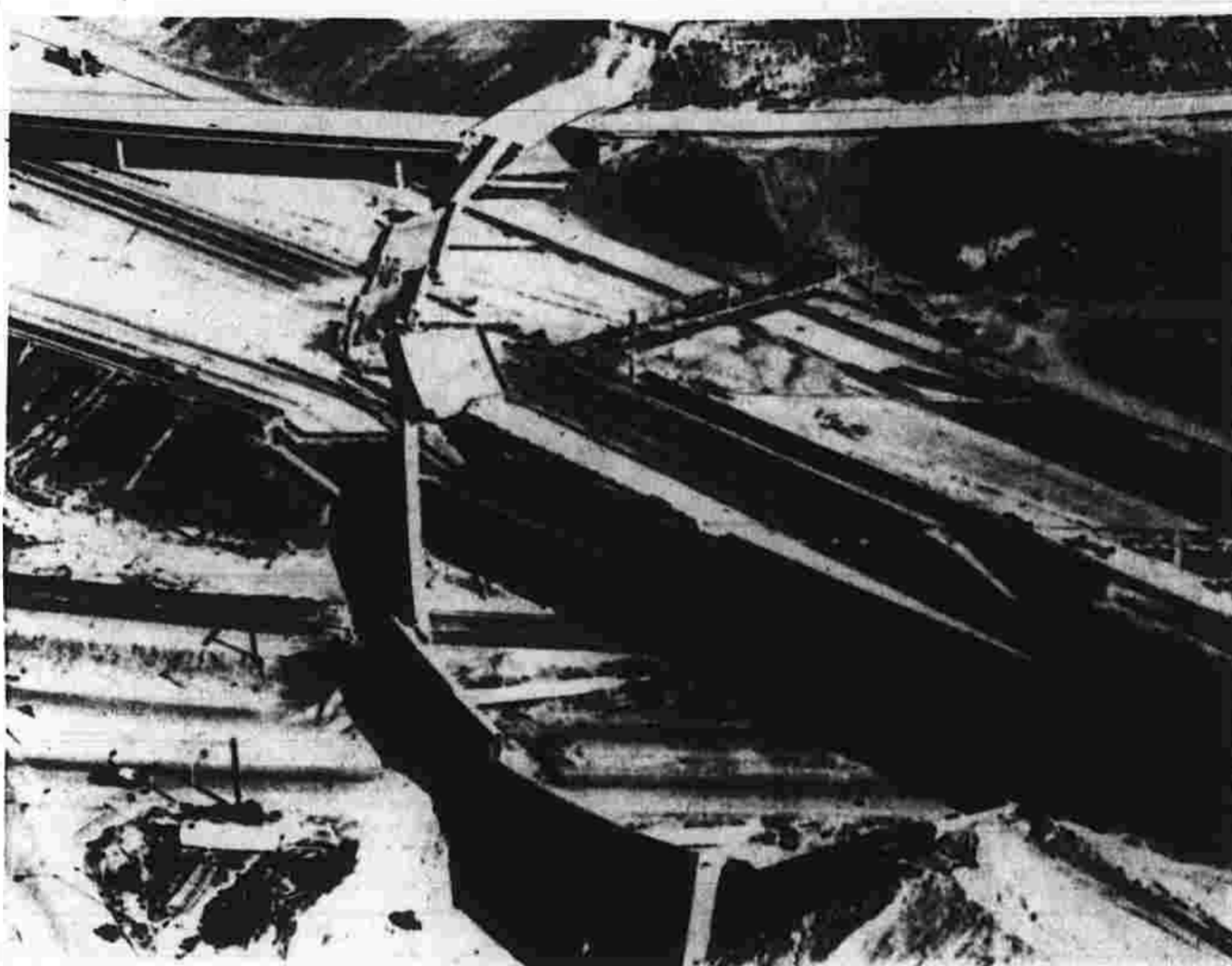
Section of overpass collapsed on Golden State Freeway
