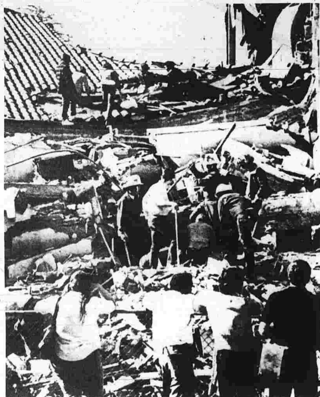
Workers dig through wreckage at VA hospital in Sylmar
